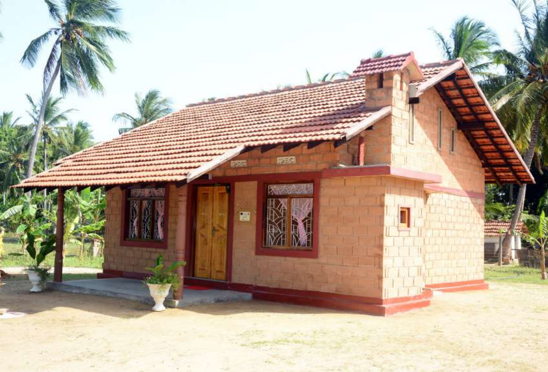
A completed house constructed through the use of appropriate technology and Earth Concrete Blocks (ECB) in Mullaitivu
