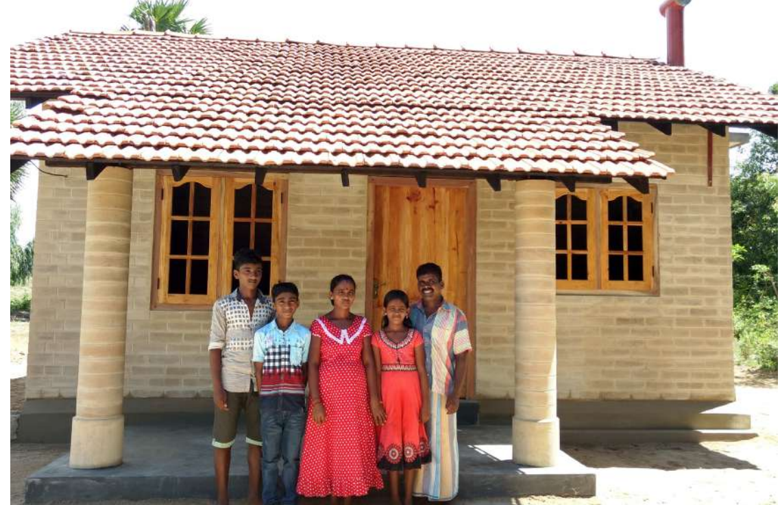
A first beneficiary family to receive a Habitat home constructed with the use of Compressed Stabilized Earth Blocks (CSEB) in Batticaloa. (Photo: Jim Kendall)
